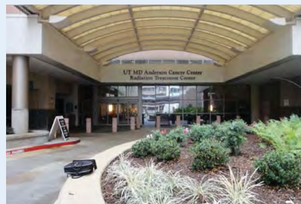
Fig.9: Radiation Treatment Center
